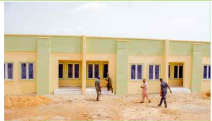
Newly constructed primary schools
