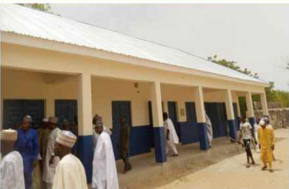
Newly constructed primary schools
