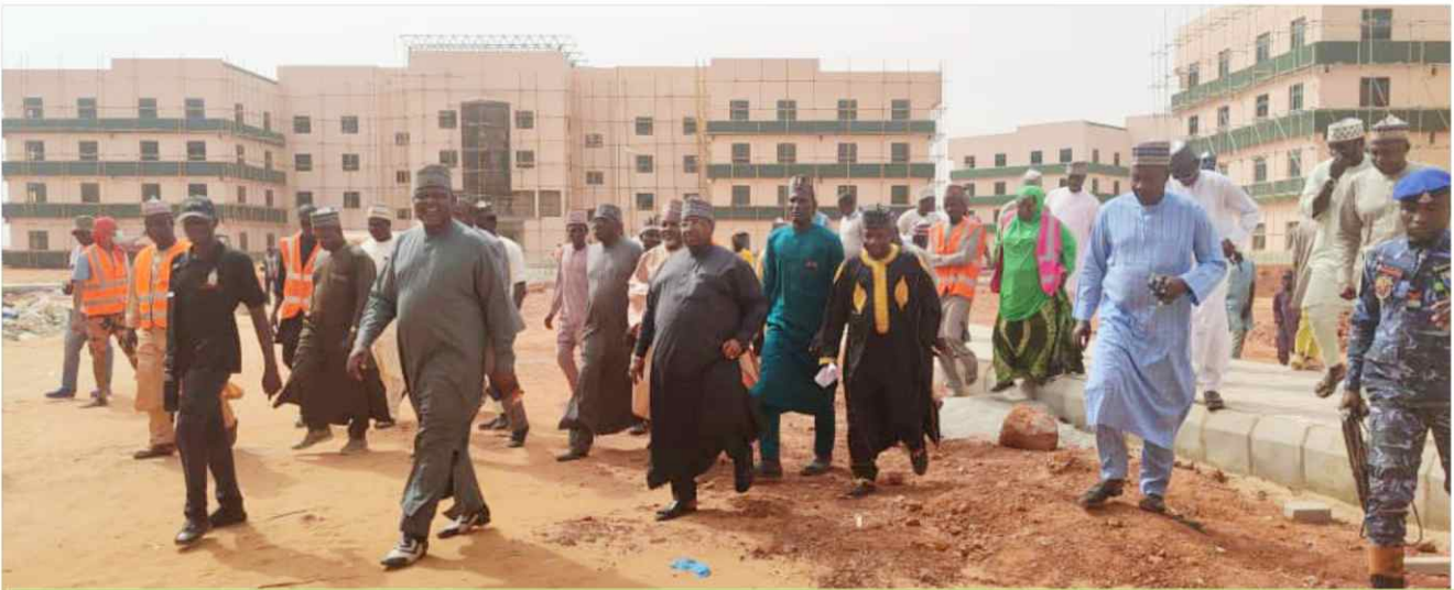
Gov Nasir Idris inspecting the ongoing construction of Ultra modern State Secretariat complex at Gwadagaji, work has reached over 80 percent completion
